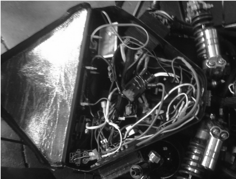
Enclosure wiring mess graphic
